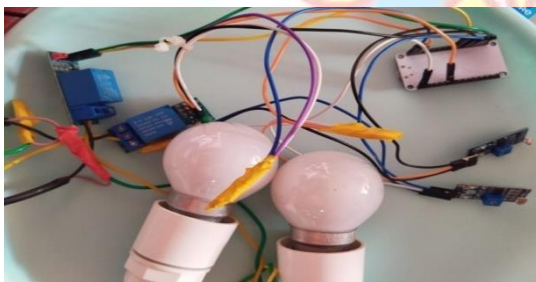
Figure 7: Connection of street light
