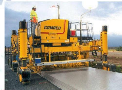
Horizontal slip forming
