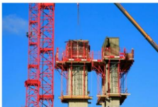
Slip form Construction Technique
