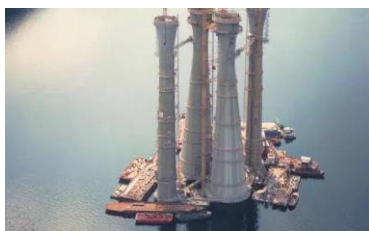
Conical slip forming
