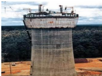
Slip Form Work Construction
