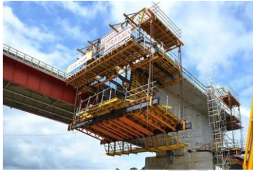
Cantilever slip forming
