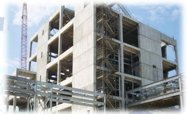
Fig 1.Reinforced concrete shear wall
