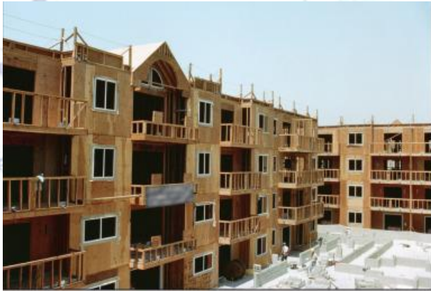
Fig 4. Plywood shear wall
