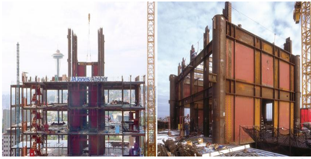
Fig 3. Steel shear wall
